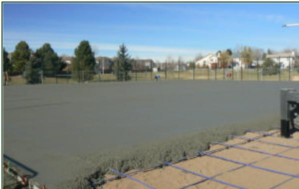
Construction began Nov. 3 with site prep and demolition of the old court. On Nov. 12, the post tensioned concrete was poured and fence posts installed.
