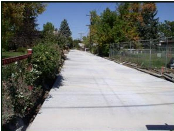
The concrete has been poured from end to end for the main alley in block 29. The remaining work includes grading the edges and placing crusher fines.
