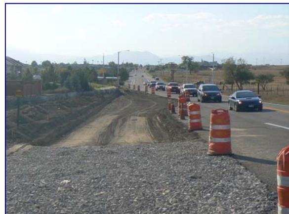
Lowell Boulevard and Shannon Drive, adding curb and gutter and edge drains between Lowell Boulevard and Shannon Drive to improve drainage, re-striping roadway between Federal Boulevard and Zuni Street to allow for a right-turn lane at McKay Park Drive, and installing of a traffic signal at the intersection with McKay Park Drive.
