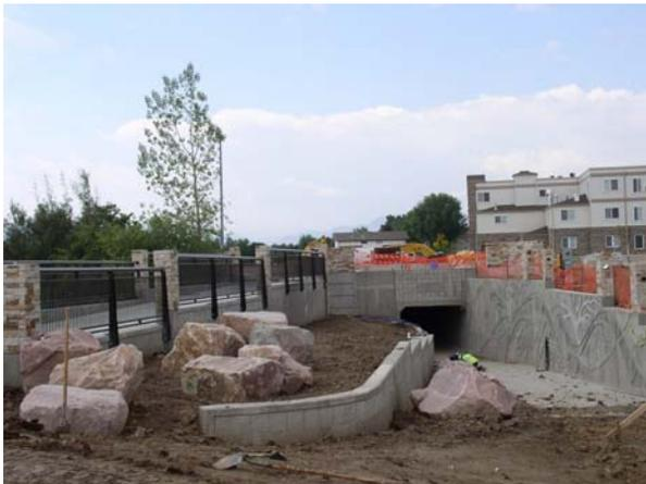
Currently, most of the work is focusing on construction of the west-side retaining walls. The east side is mostly complete except for landscaping and installation of the remaining handrails. Old and broken concrete along Sheridan Boulevard has been replaced and the final layer of asphalt has been paved. Qwest Communications is in the process of relaying their communication lines along the west side of Sheridan.
