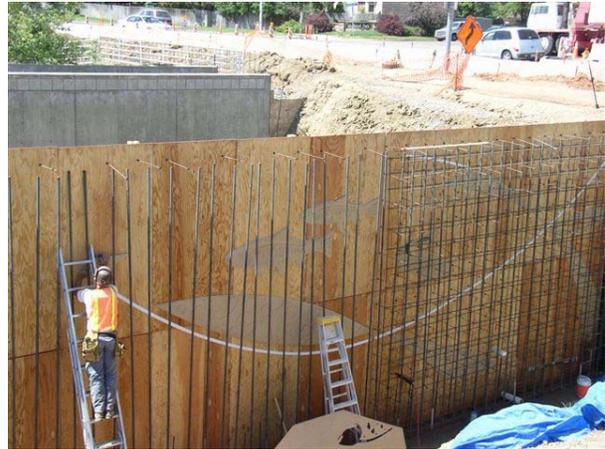
**The contractor continues to construct concrete retaining walls on the east side of Sheridan for the underpass.**
