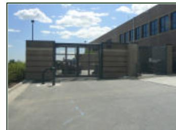
The Sally Port improvements added structural masonry walls and detention-grade security gates to the exterior of the north side of the Police/Courts Building at 17 DesCombes Drive. This created a 2,670 square foot secure outdoor space to allow detainee transfers to be completed in a secure and private area.
