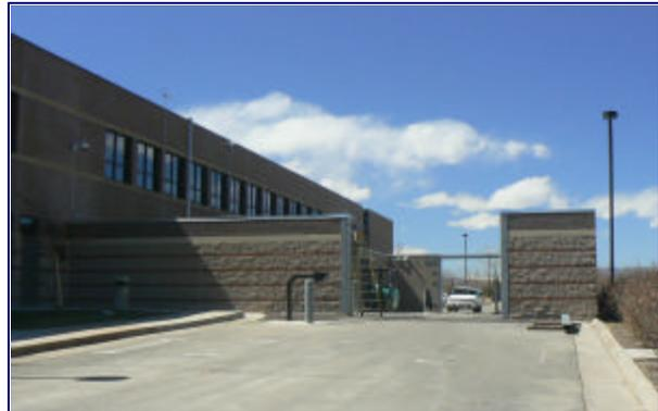
Haselden Construction has finished all major structural and security components of the sally port. Final painting of the metalwork will be scheduled when the weather is warmer and dryer. The specialty security doors have been ordered and will be delivered in late April. They will be installed and painted and the sally port will be substantially complete. Training and testing will occur throughout the month of May.
