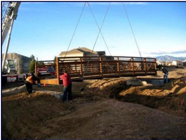
currently being fabricated. The bridge over Community Ditch was lifted into place on Jan. 8, and the concrete approaches will be poured as weather allows.
